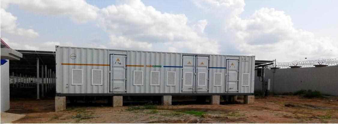
Diesel/PV/battery hybrid microgrid system in South Sudan
