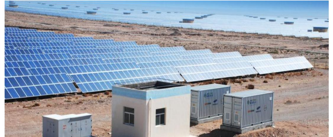
The first DC coupled battery storage system to solve the PV curtailment
